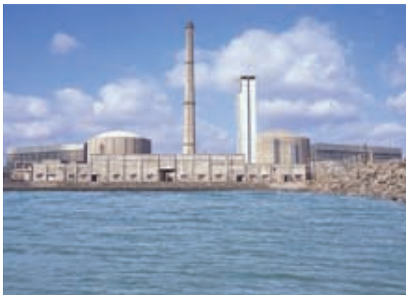
Tarapur Atomic Power Project Unit - 3 & 4 (2x540) MWe, Thane Dist., Maharashtra
