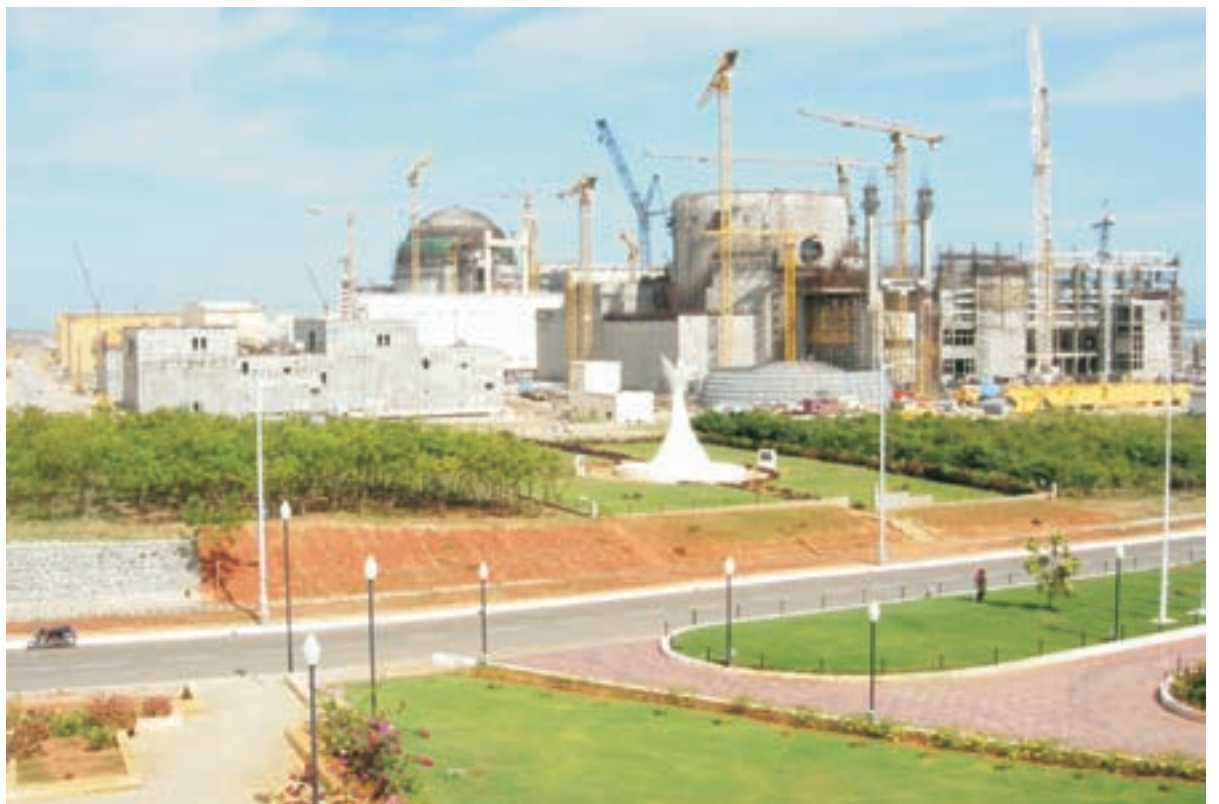
Kudankulam Atomic Power Project Unit - 1 & 2 (2x1000) MWe, Tirunelveli Dist., Tamil Nadu
