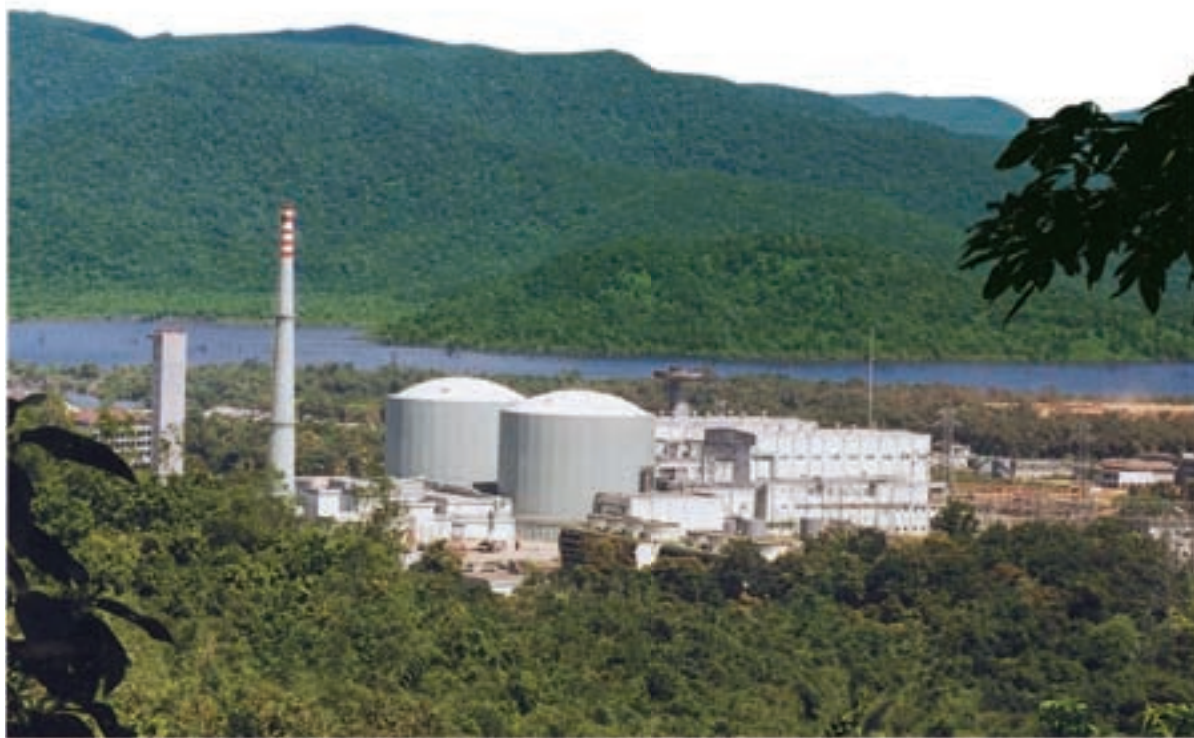
Kaiga Atomic Power Station Unit - 1 & 2 (2x220) MWe, Uttar Kanada Dist., Karnataka
