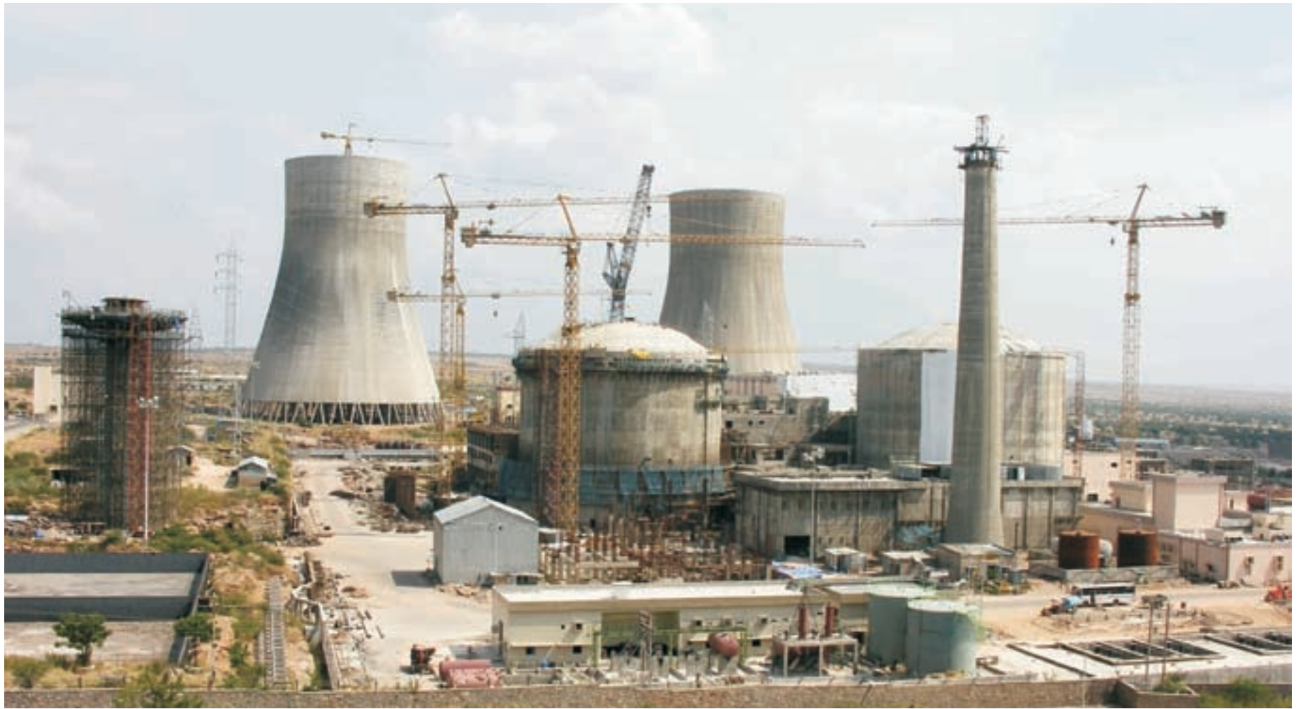
Rajasthan Atomic Power Project - Unit 5 & 6 (2x220) MWe, Chittorgarh Dist., Rajasthan
