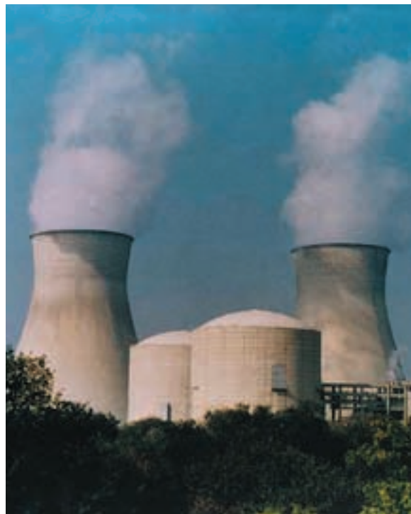
Above: Narora Atomic Power Station Unit - 1 & 2 (2x220) MWe, Bulandshahr Dist., Uttar Pradesh
