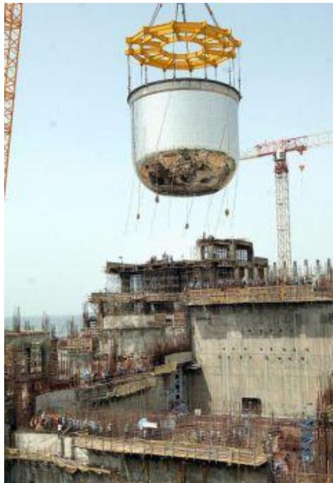
**The safety vessel, one of the major nuclear reactor components, being lowered into the reactor vault at the Indira Gandhi Centre for Atomic Research, Kalpakkam. A file picture.**
