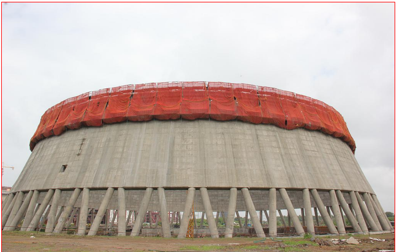
NDCT Construction work in progress
