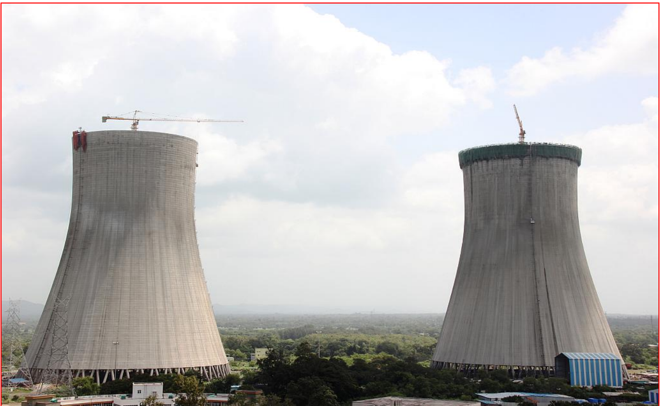
Completed shell structure of Both NDCT-3A & 3B
