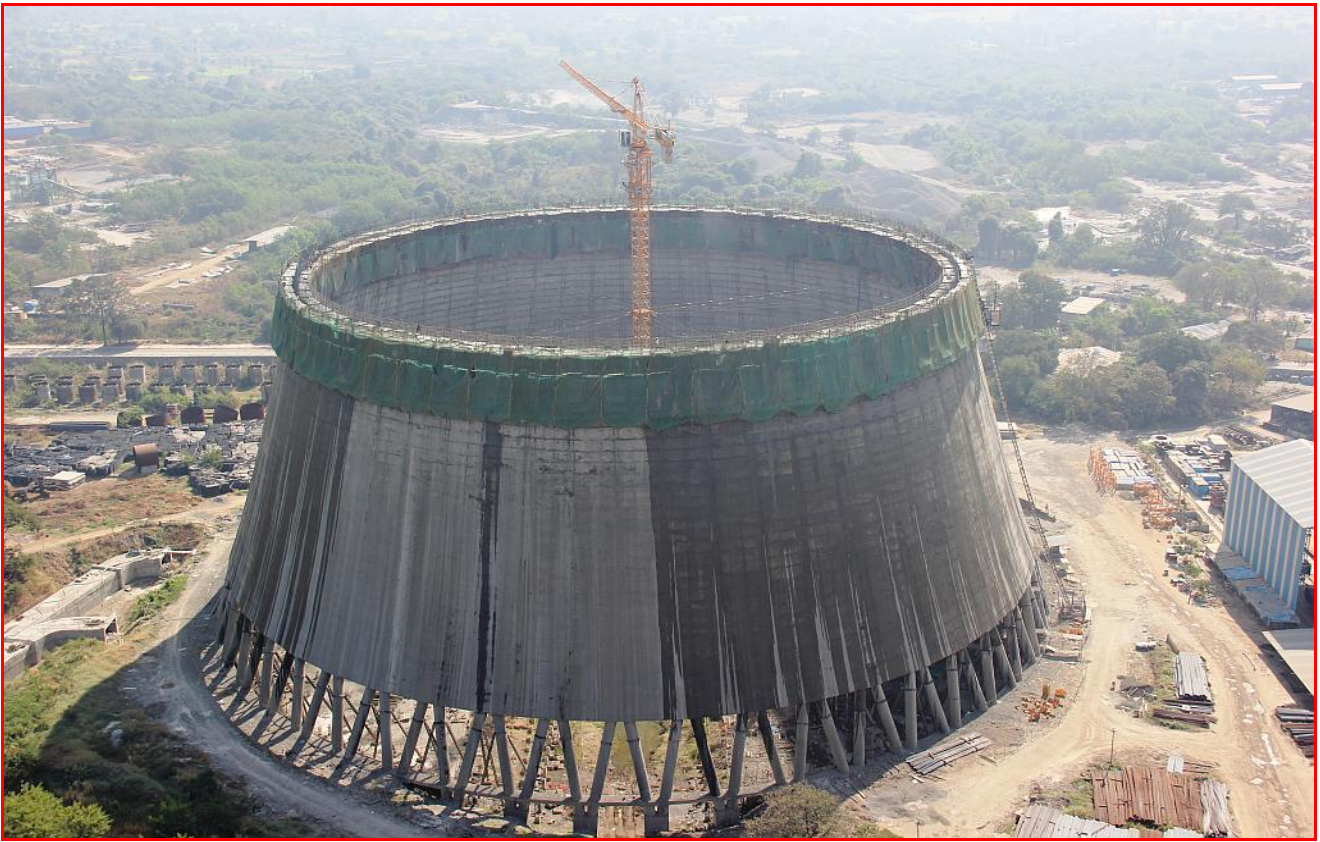
NDCT shell structure work in progress
