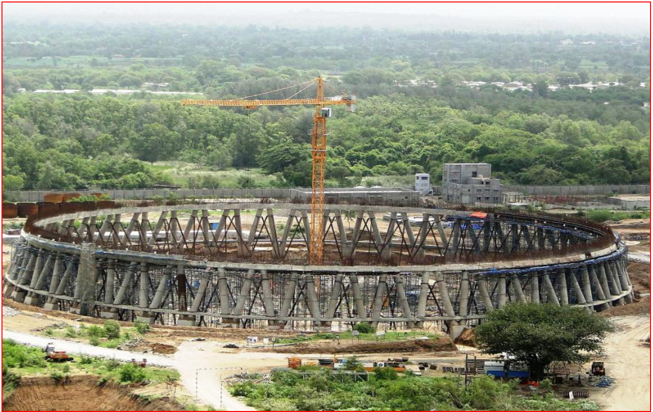
NDCT Construction work in progress
