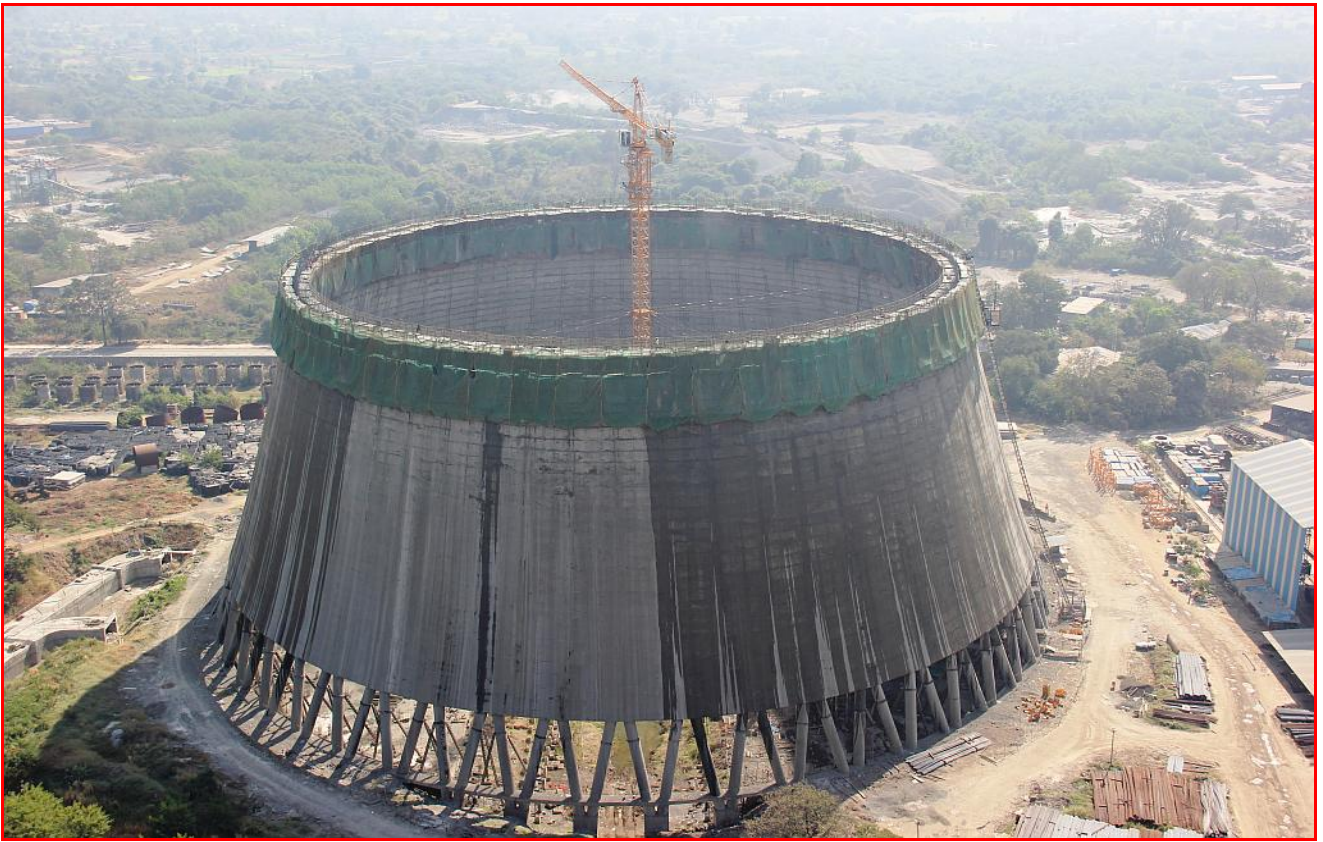
NDCT#3B shell structure
