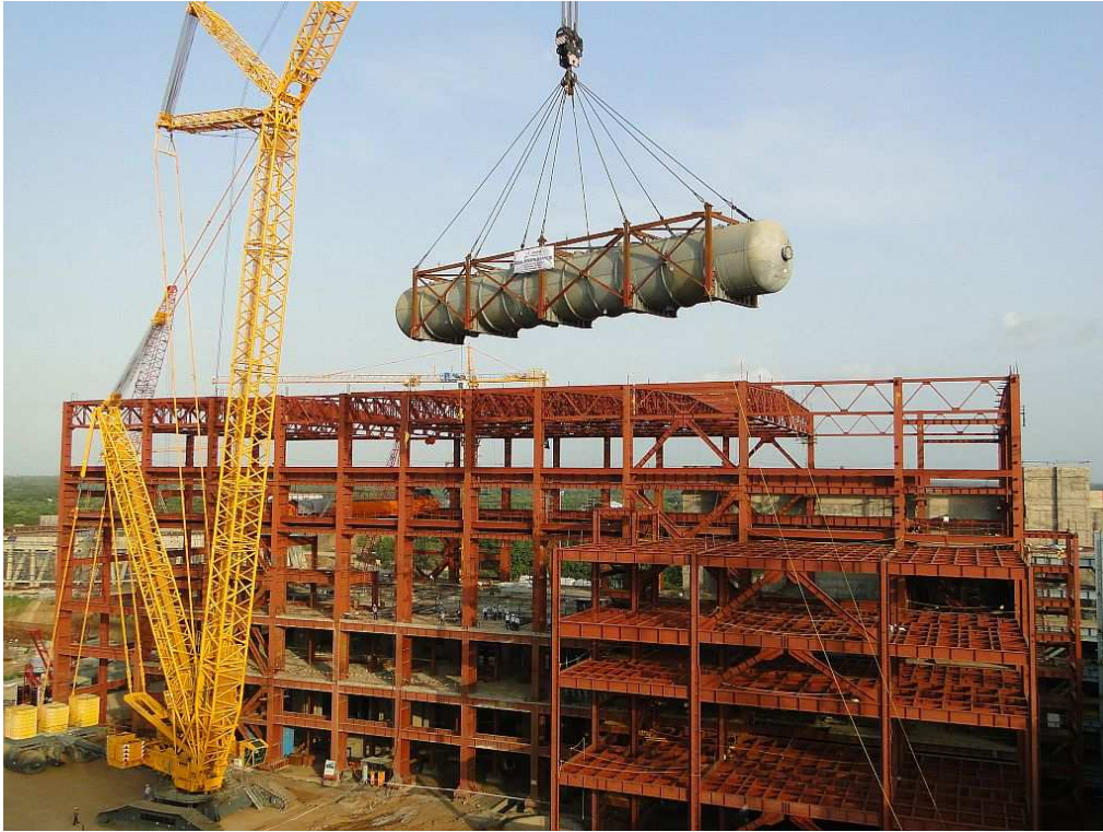
Deaerator Storage Tank Erection in TB-3
