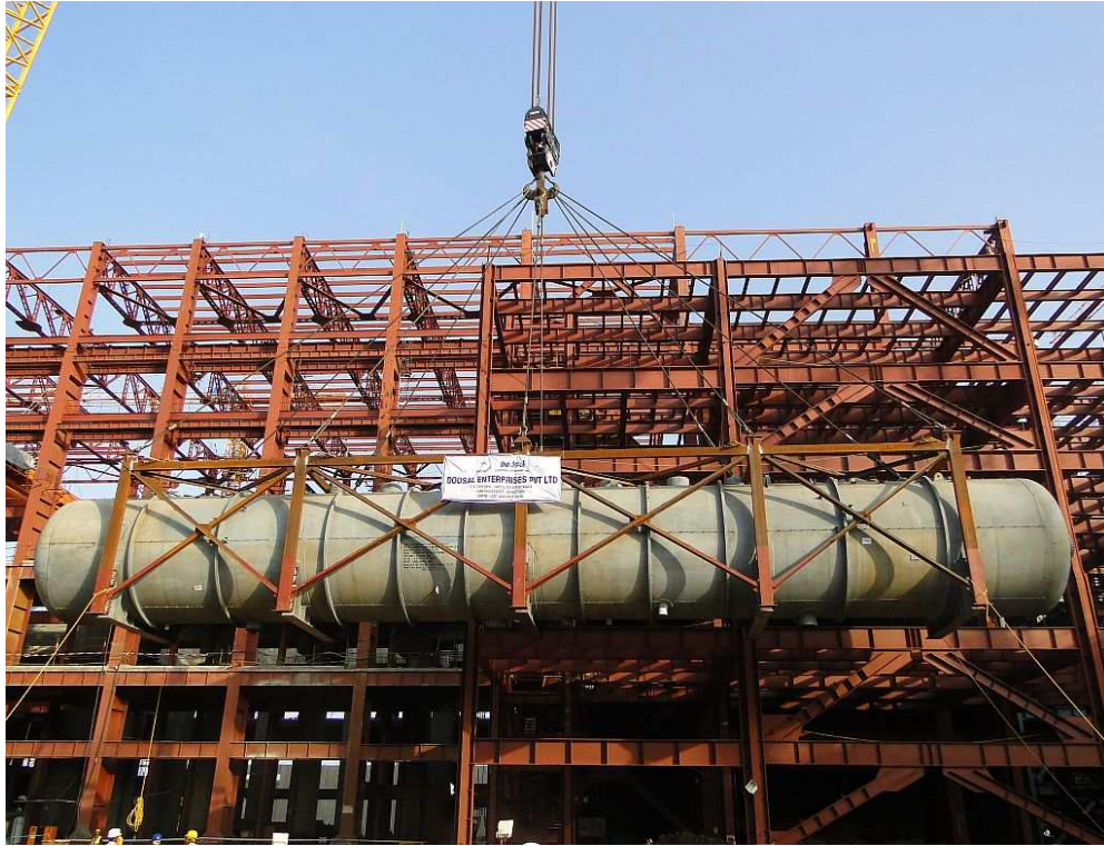
Deaerator Storage Tank Erection in TB-3
