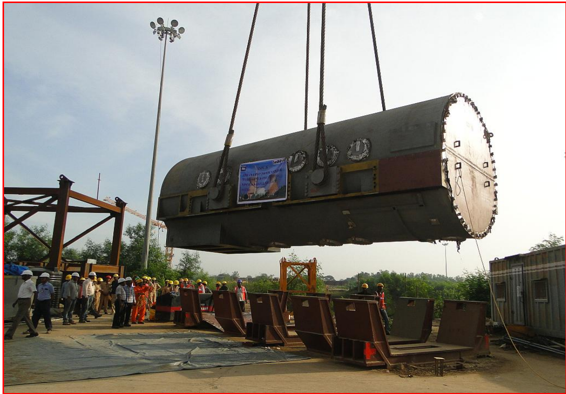
Generator Stator Erection in TB-3
