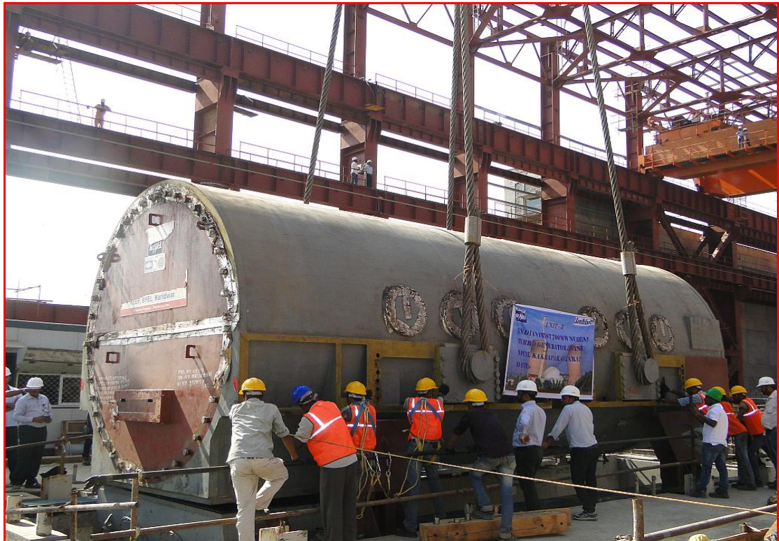
Generator Stator Placement in TG#3 deck at EL 118 M
