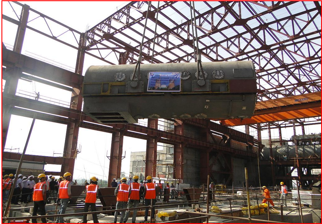
Generator Stator Placement in TG#3 deck at EL 118 M
