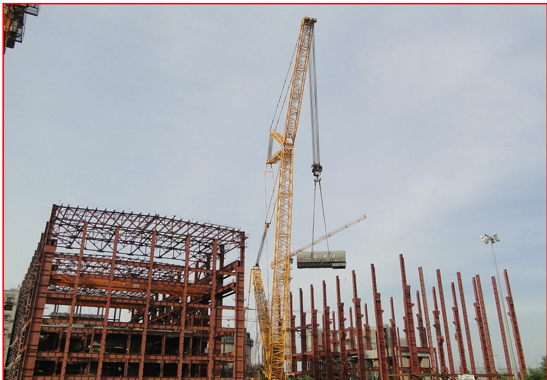
Generator Stator Erection in TB-3
