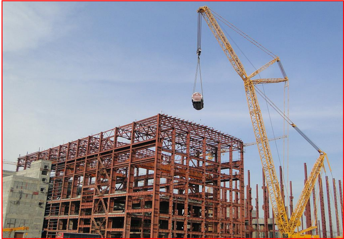
Generator Stator Erection in TB-3
