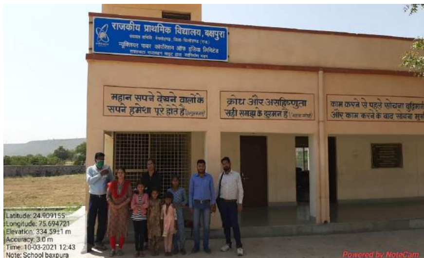
School building construction at Bakshpura
