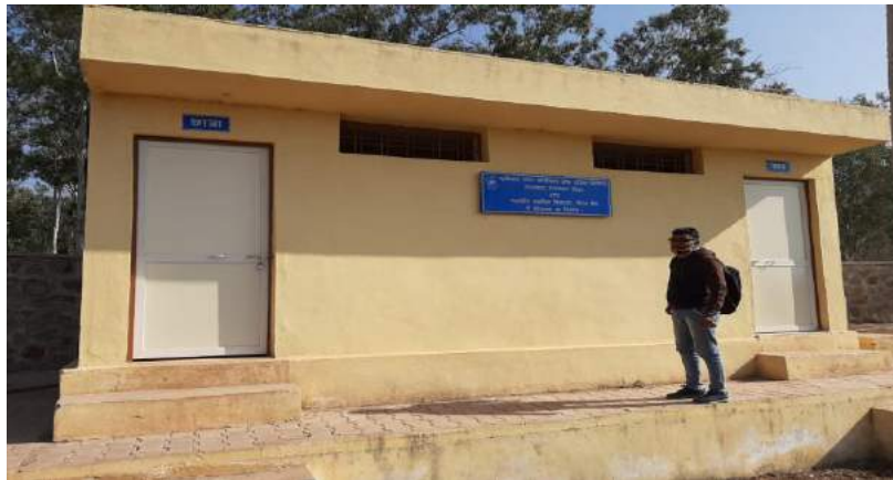
Toilet constructed at PS, Sedal Dam
