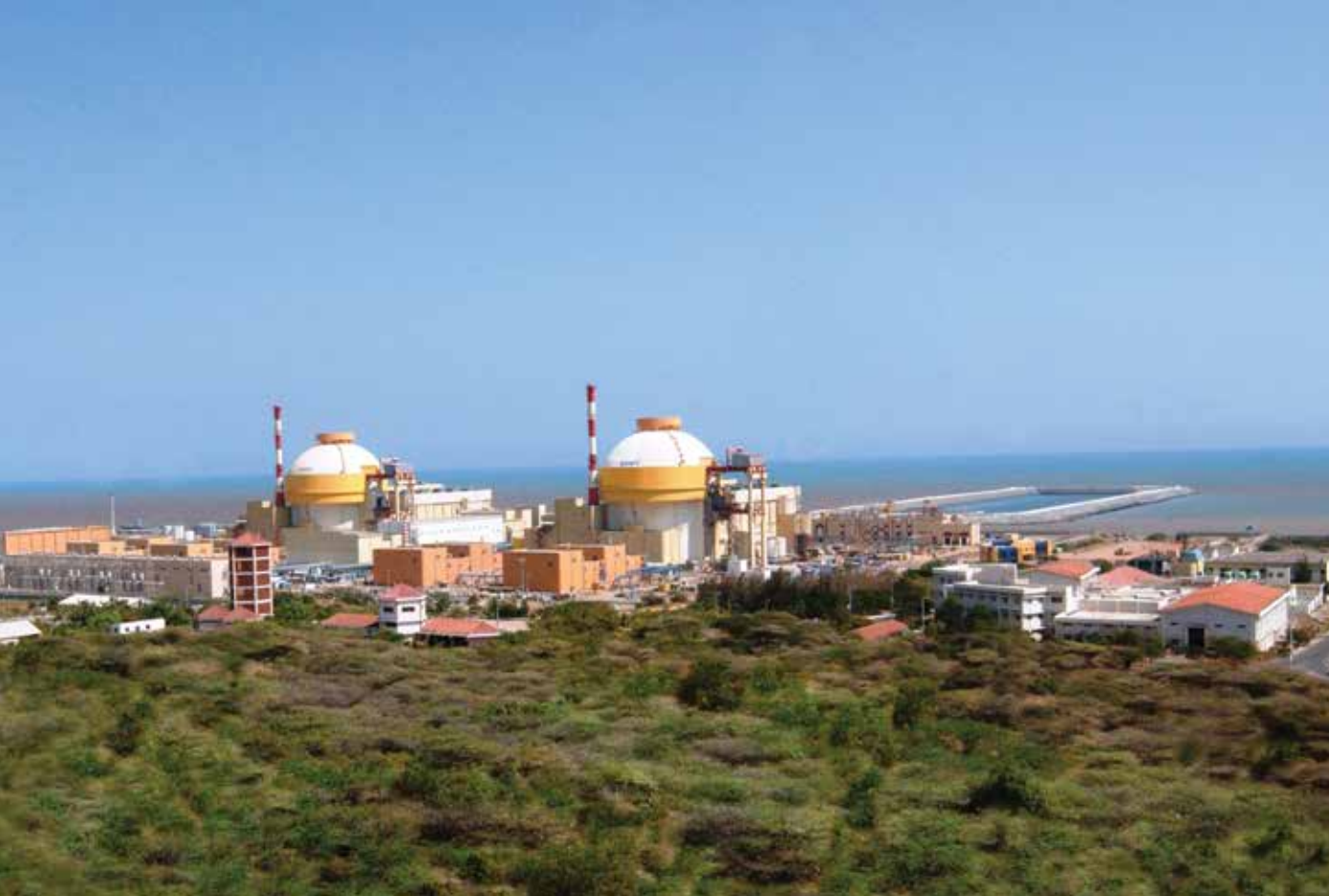
Kudankulam Nuclear Power Project
