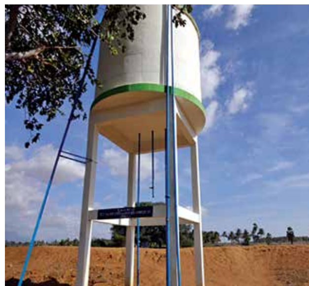
Construction of water tank in Radhapuram near Kudankulam in Tamil Nadu
