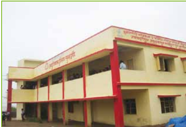
Construction of Anuvikas School in the neighbourhood of Tarapur, Maharashtra as part of CSR initiative.
