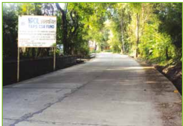
Construction of Chinchani Varor Road in the neighbourhood of Tarapur, Maharashtra as part of CSR initiative in Infrastructure Sector.
