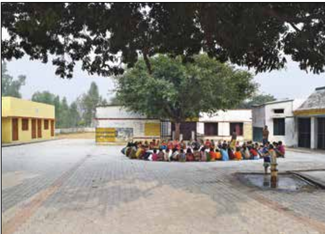
Construction of Class Rooms and Flooring at a School near Narora, Uttar Pradesh
