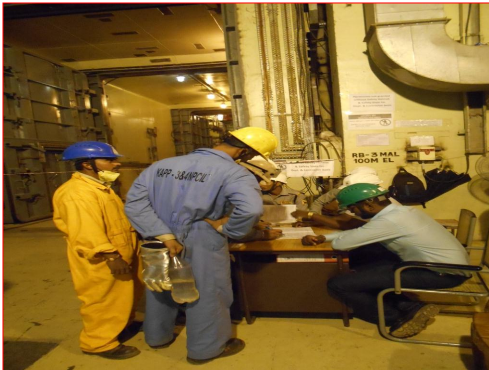
Access control in RB-3 during Hot Conditioning
