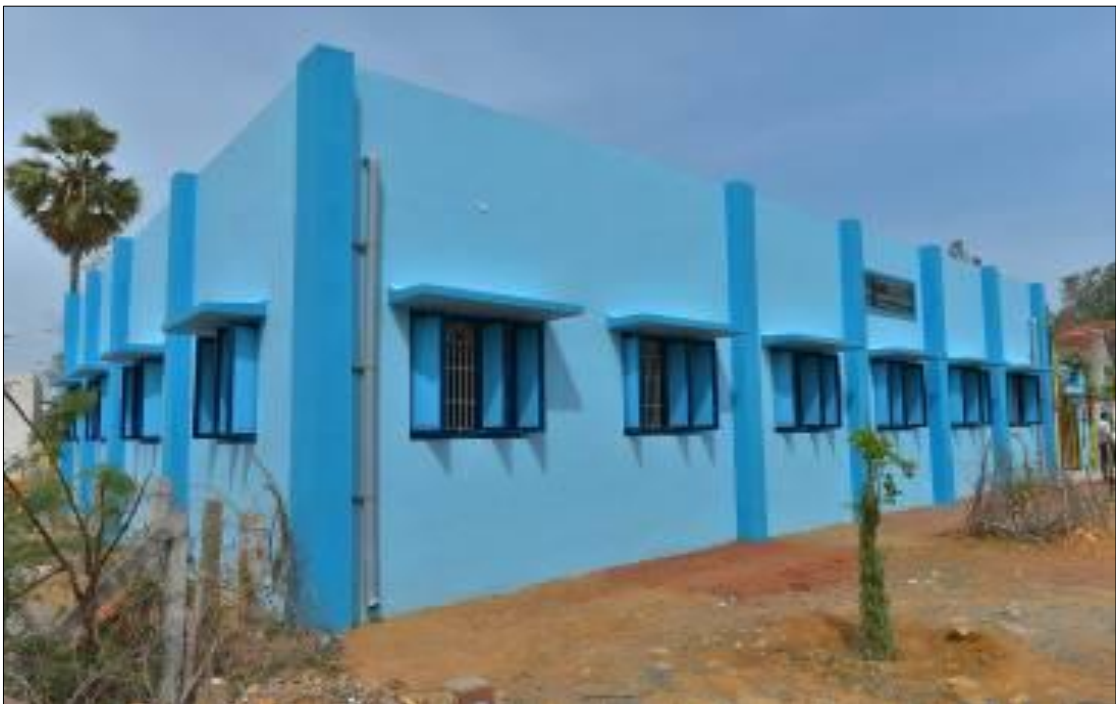
Construction of additional class room building at Parameshwarapuram, Tamil Nadu
