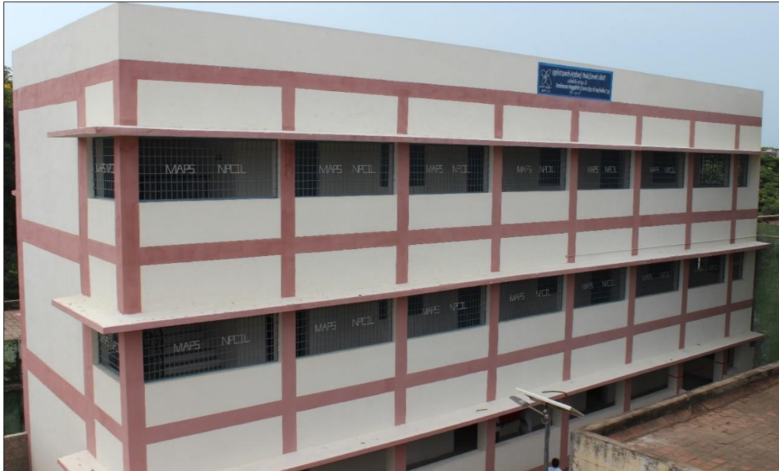
Construction of Government Higher Secondary School at Pudupattinam, Tamil Nadu
