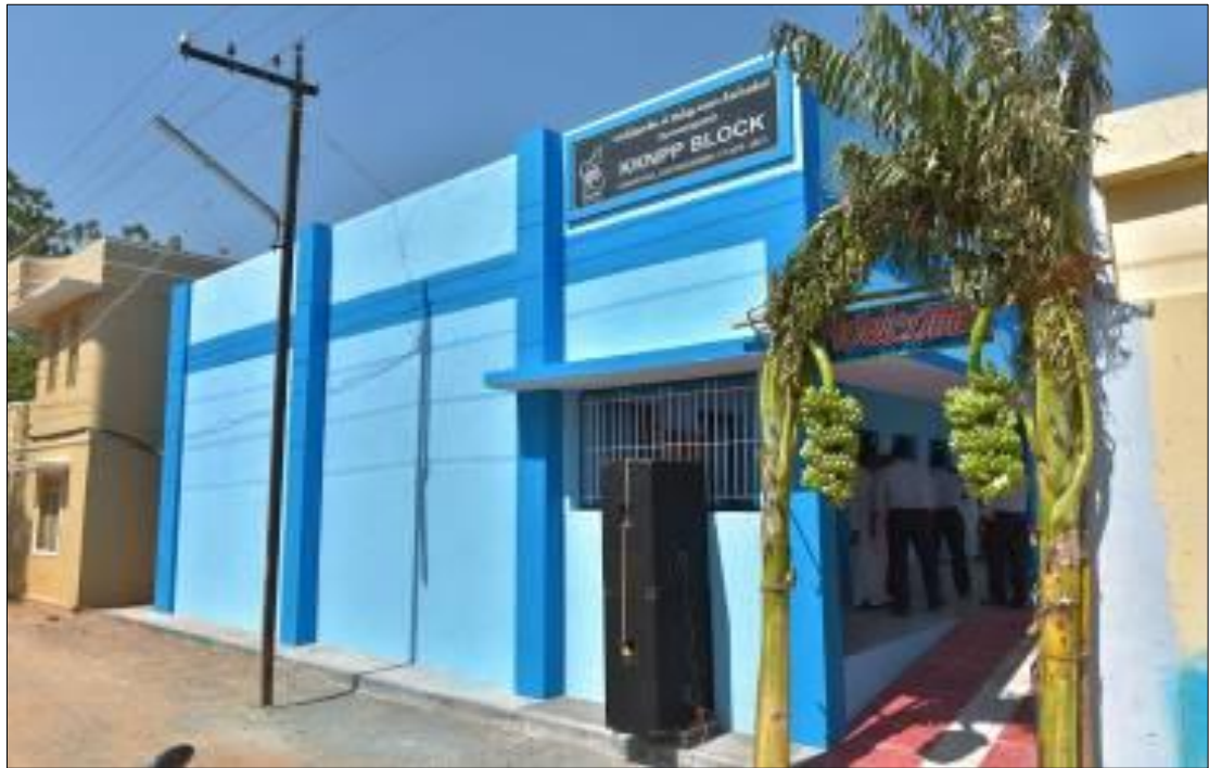
Construction of additional class room building with furniture at Avaraikulam, Tamil Nadu
