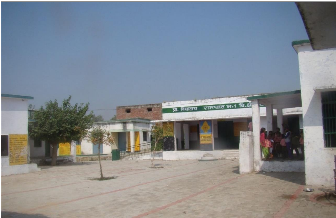
Construction of open ground development at Prathmic Vidyalaya, Ramghat, Uttar Pradesh
