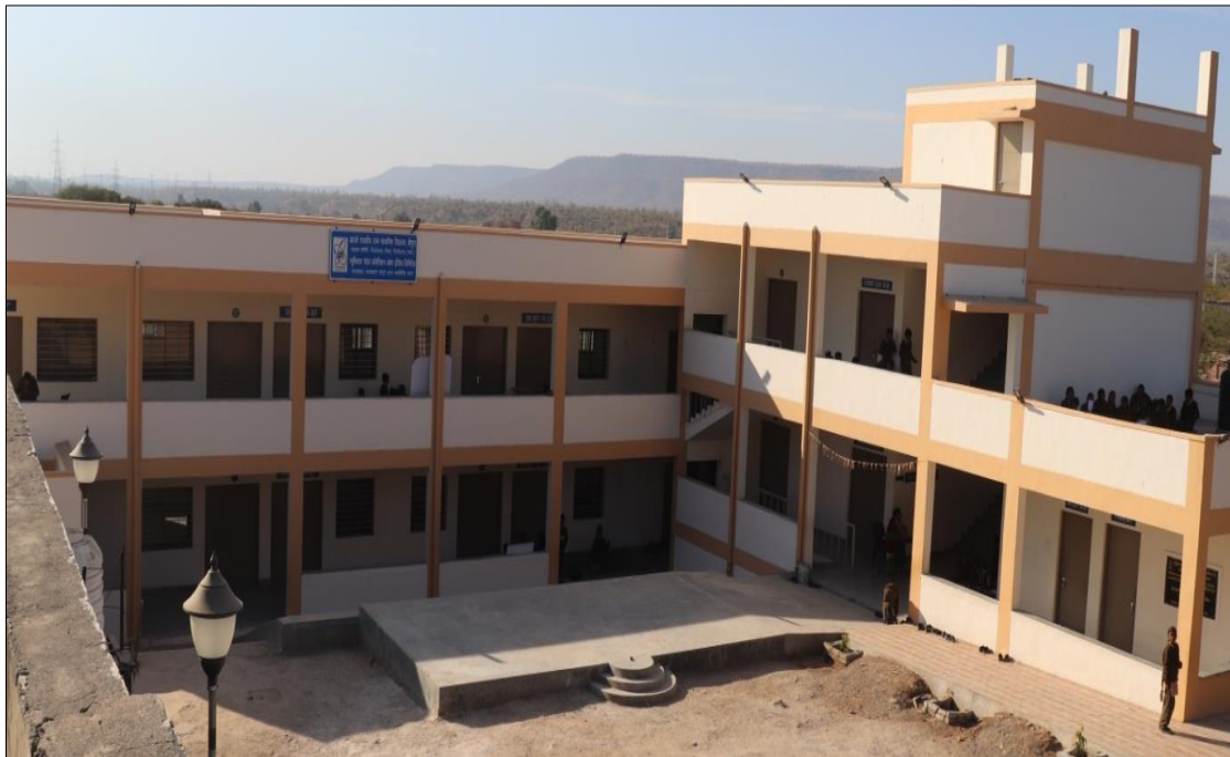
Construction of Government Senior Secondary School at Shripura, Rajasthan
