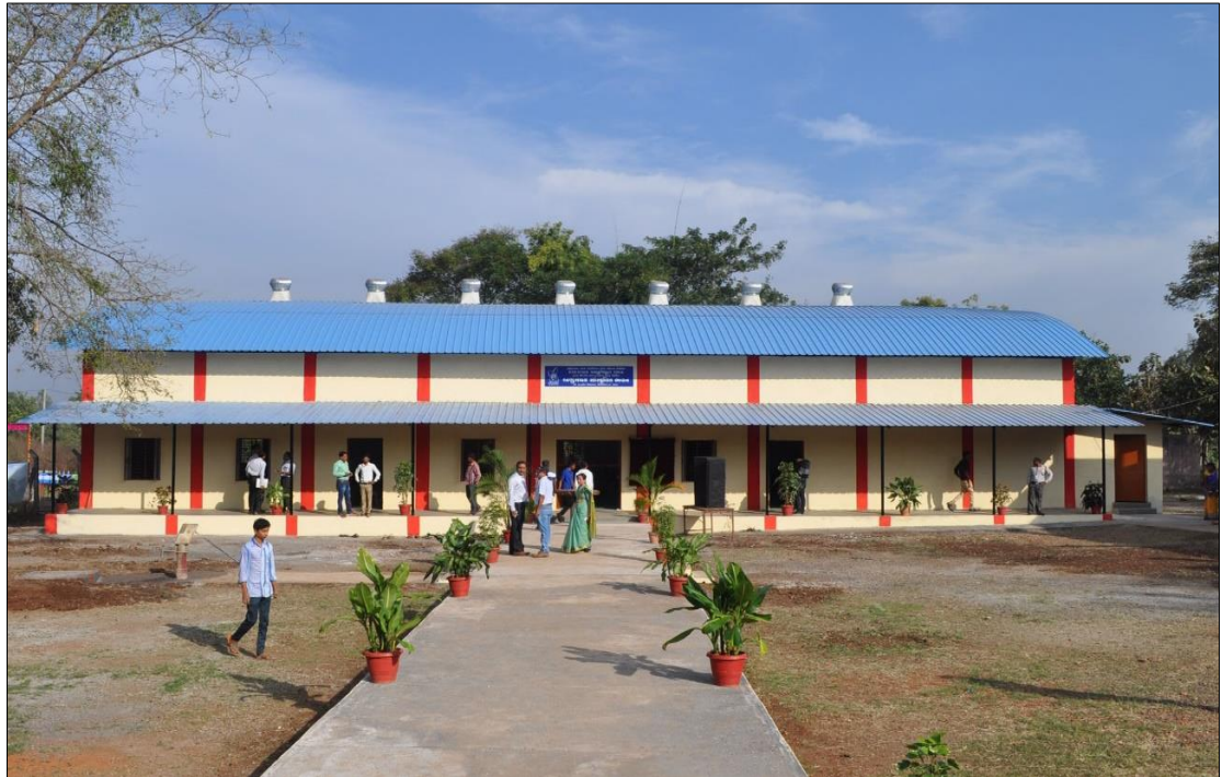
Construction of Anumathak Sanskritik Bhavan at Unchamala School, Gujarat
