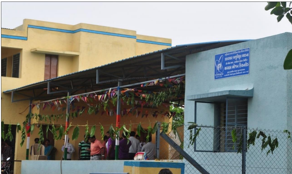
Construction of Kitchen & mid-day meal shed at Juna Kakrapar, Gujarat
