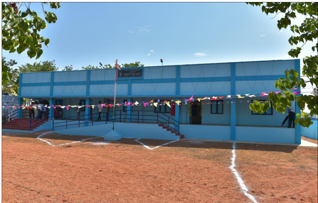
Construction of additional class room building with furniture at Dhanakkarkulam, Tamil Nadu
