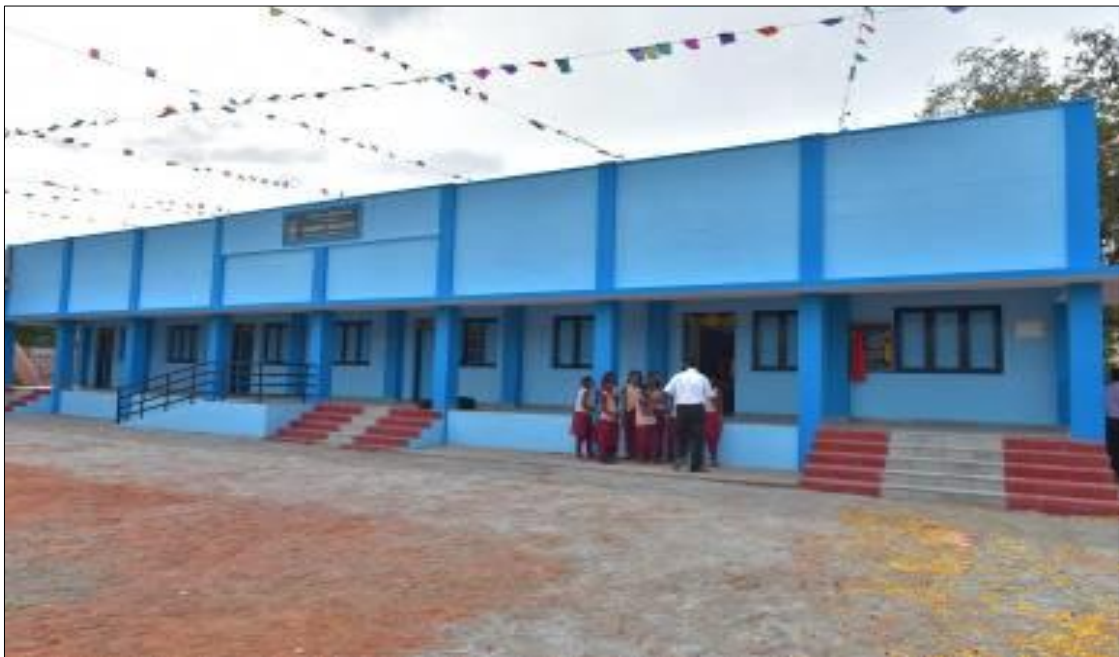
Construction of additional class room building with furniture at Vadakkankulam, Tamil Nadu
