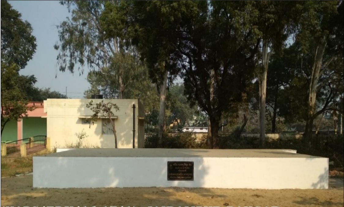
Construction of platform for flag hoisting at Inter College, Narora, Uttar Pradesh
