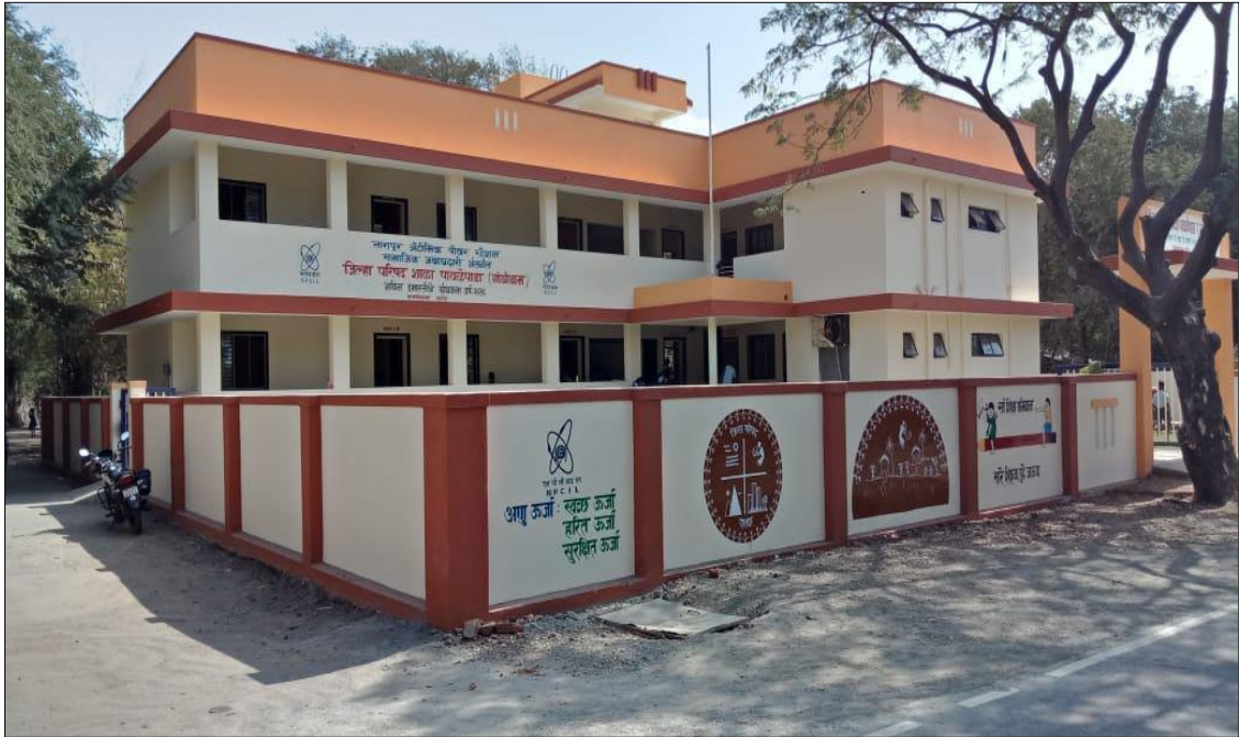
Construction of Primary School at Gandhidham, Maharashtra
