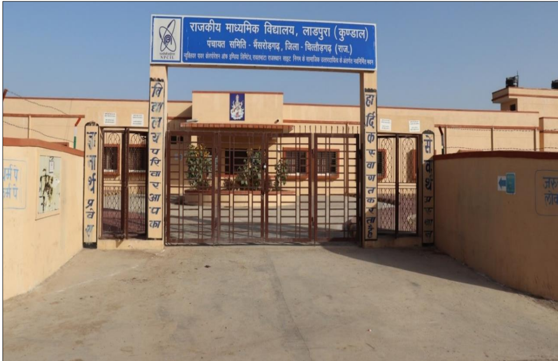
Construction of Government Higher Secondary School at Ladpura, Rajasthan
