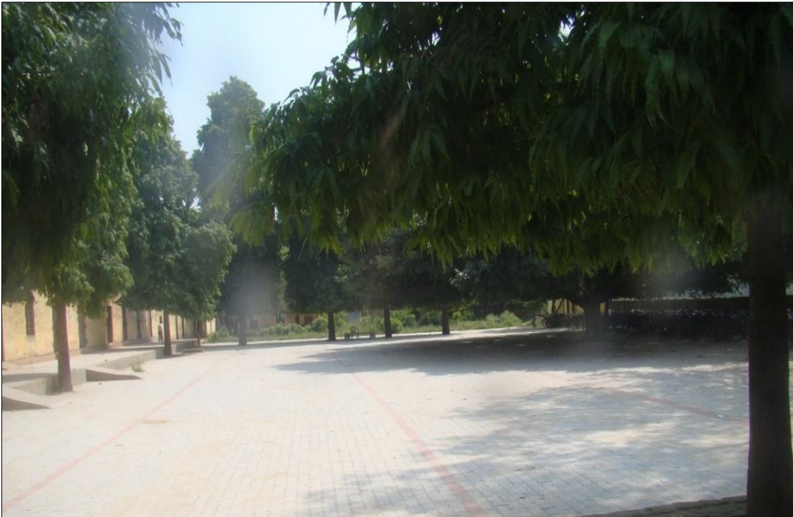
Construction of open area flooring at Inter College, Belon, Uttar Pradesh
