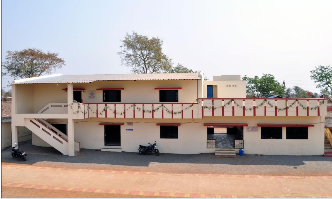
Construction of Girls Hostel at Ashramshala, Sathvav, Gujarat
