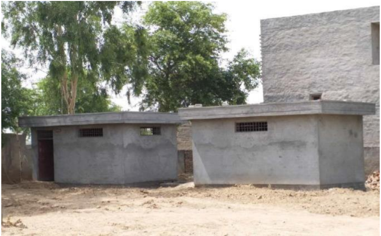
Construction of toilet blocks at Gorakhpur, Haryana
