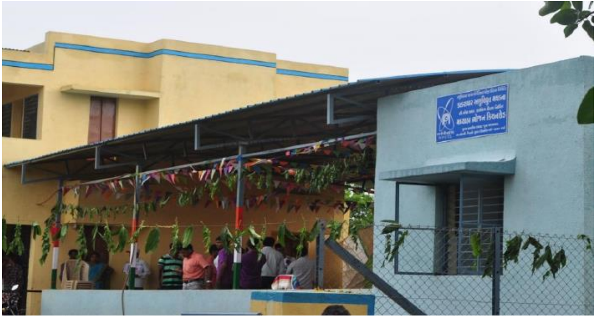
Construction of toilet block and Kitchen shed at Juna Kakrapar, Gujarat
