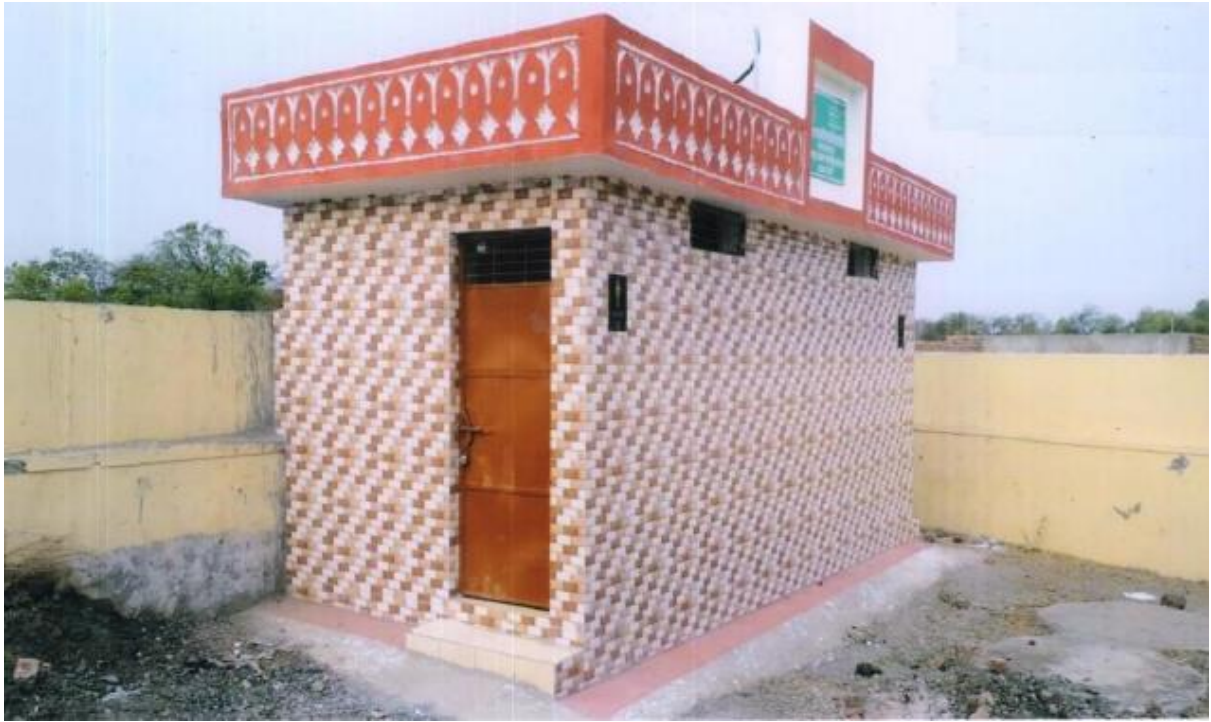
Construction of toilet blocks at Banswara, Rajasthan
