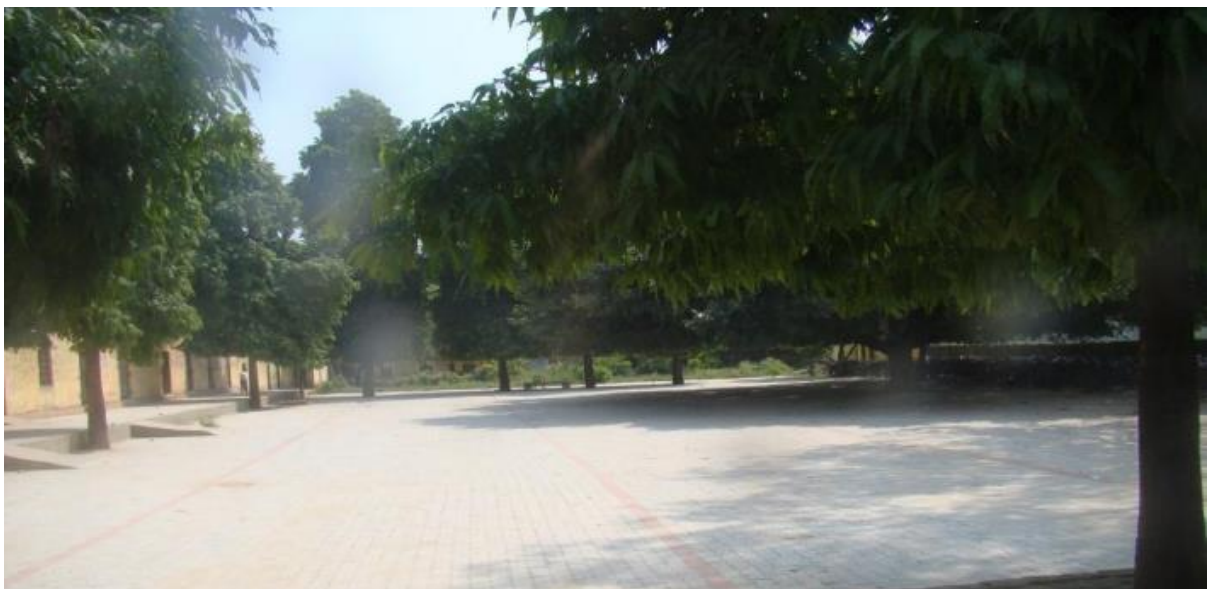
Construction of toilet block and open area flooring, Belon, Uttar Pradesh
