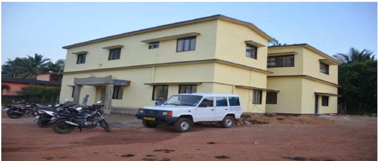
Renovation of Mallapur Health Centre, Karnataka
