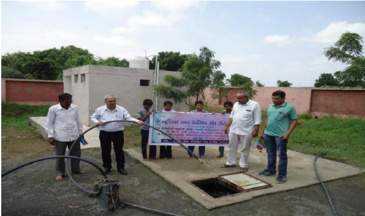
Installation of bore well at Bhavanipura, Gujarat
