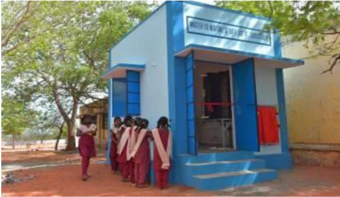
Installation of RO Plant at 3 schools near Kudankulam, Tamil Nadu
