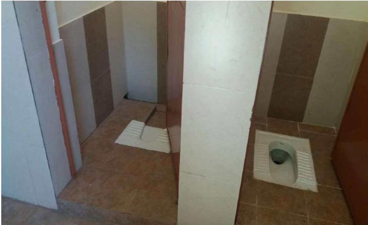
Construction of toilets at Government Schools near Rawatbhata, Rajasthan
