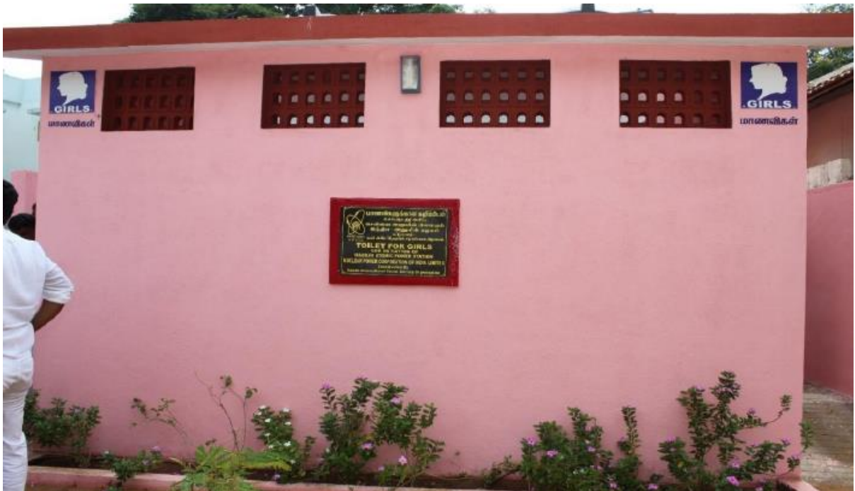
Sanitation facility at Government Schools, near Kalpakkam, Tamil Nadu
