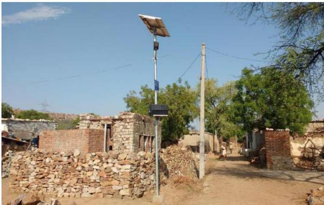
Installation of solar street lights near Rawatbhata, Rajasthan
