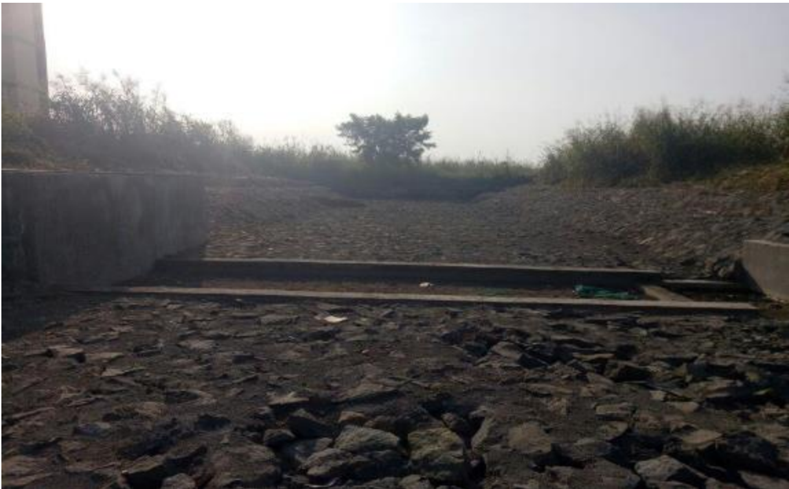
Rain water harvesting at Tarapur, Maharashtra
