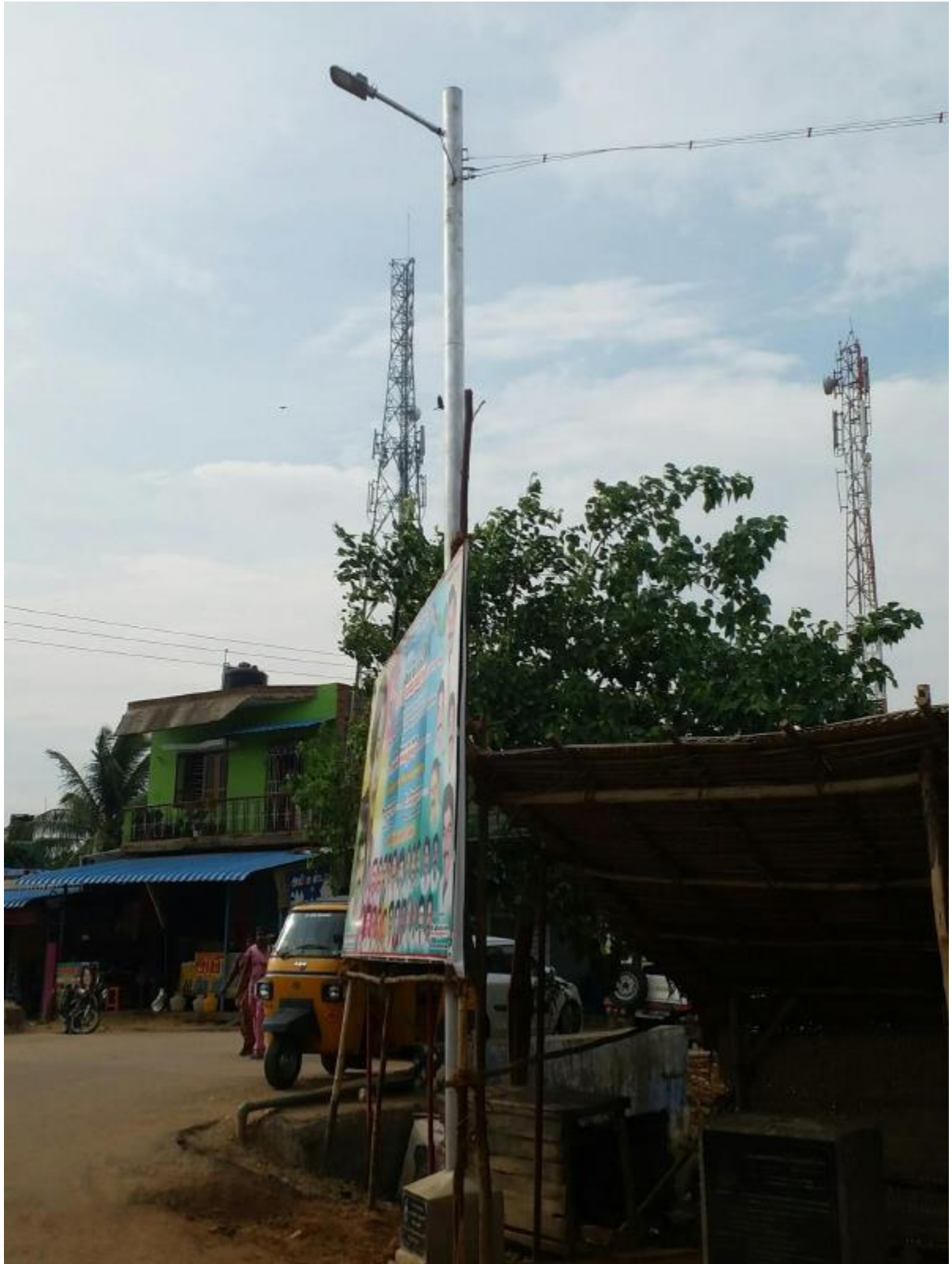
Installation of LED lights at Kudankulam
