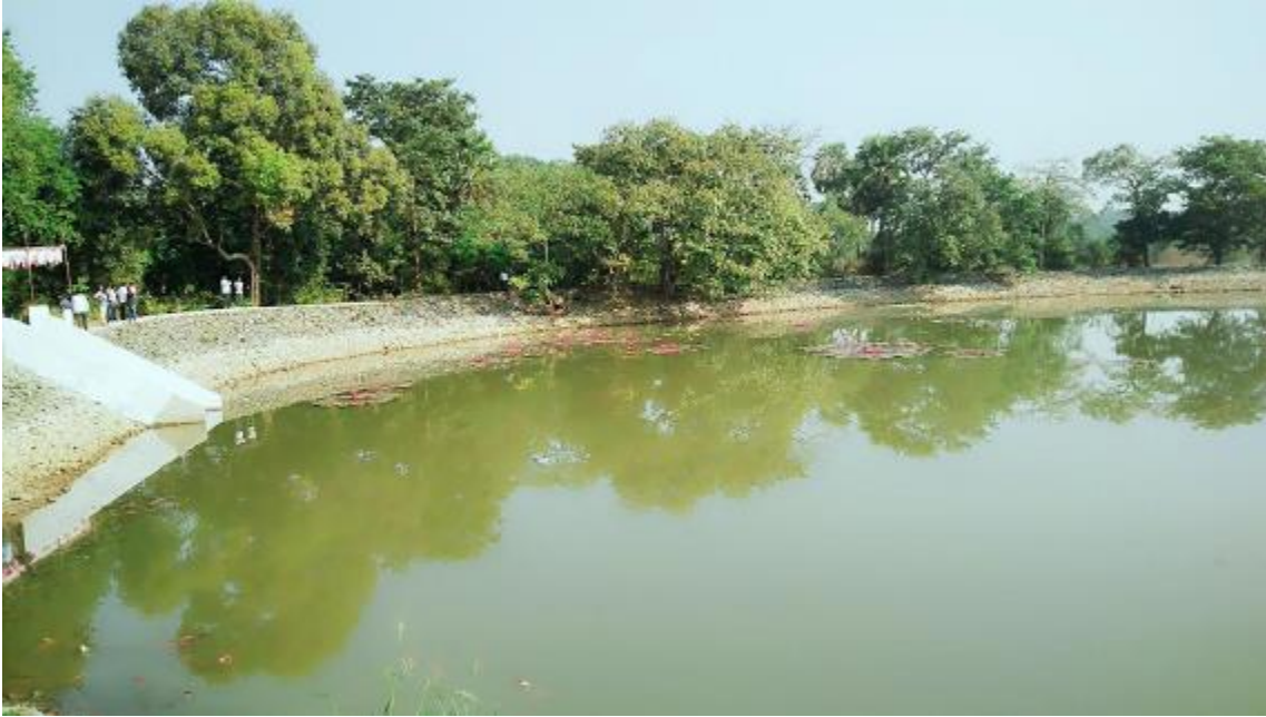
Construction of water pond at Tembhi, Maharashtra
