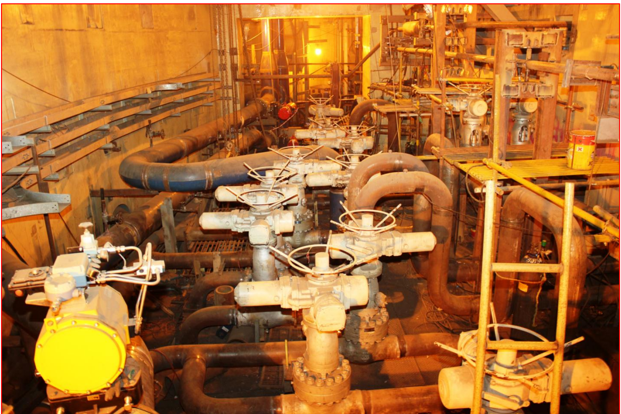
Unit#3 PHT Circuit piping work
