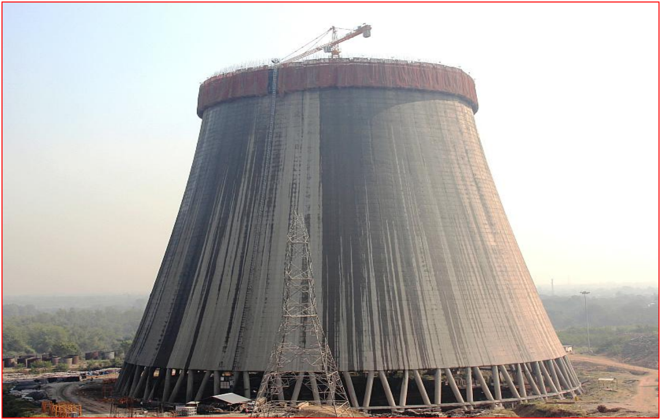
NDCT#3A construction (Nov-2016)
