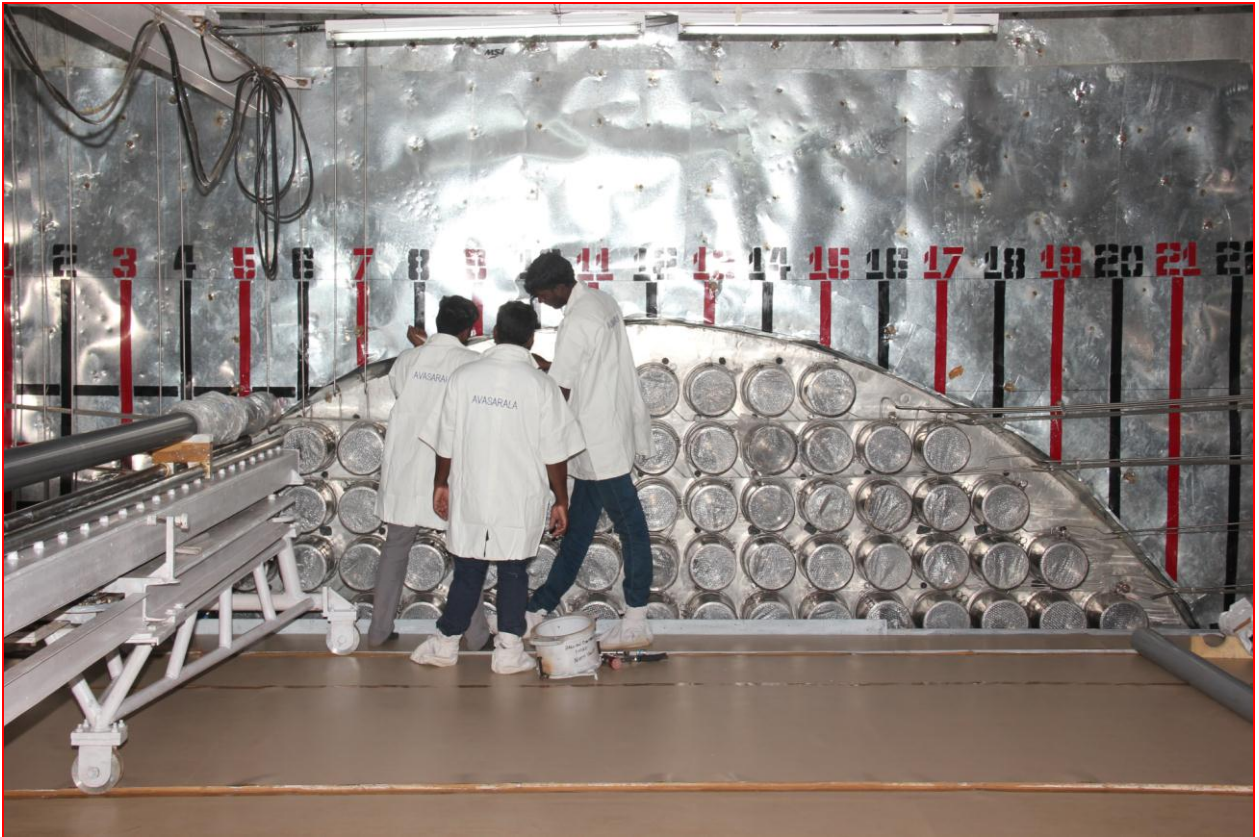
KAPP-4 Coolant Channel Installation started
