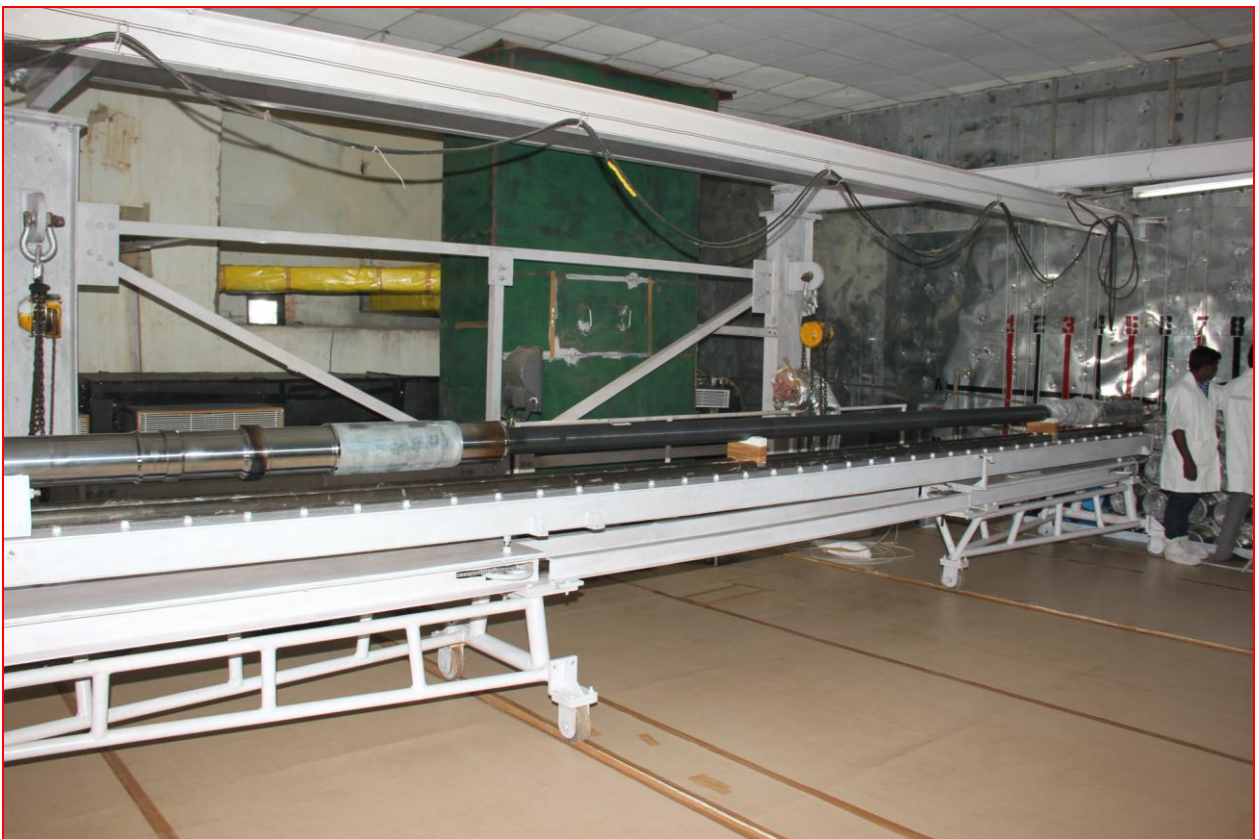
KAPP-4 Coolant Channel Installation started
