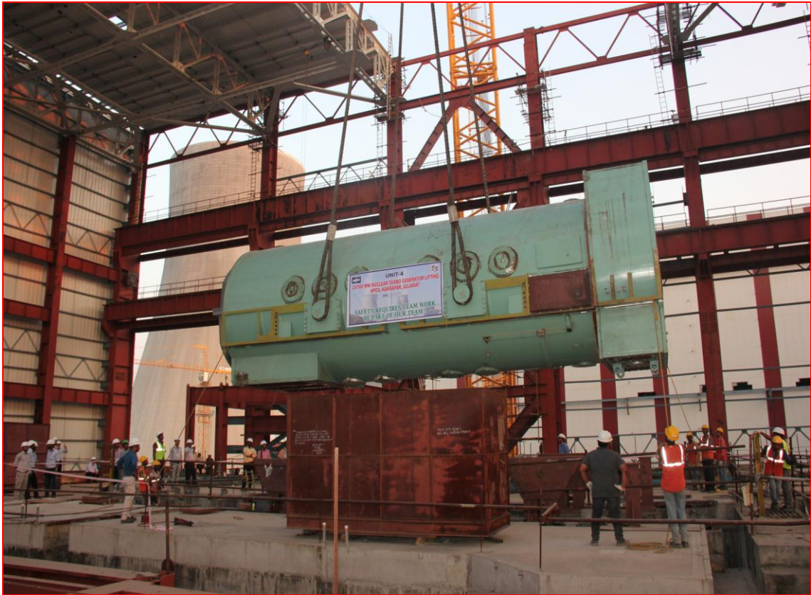
Generator Stator Placement in TG#4 deck at EL 118 M
