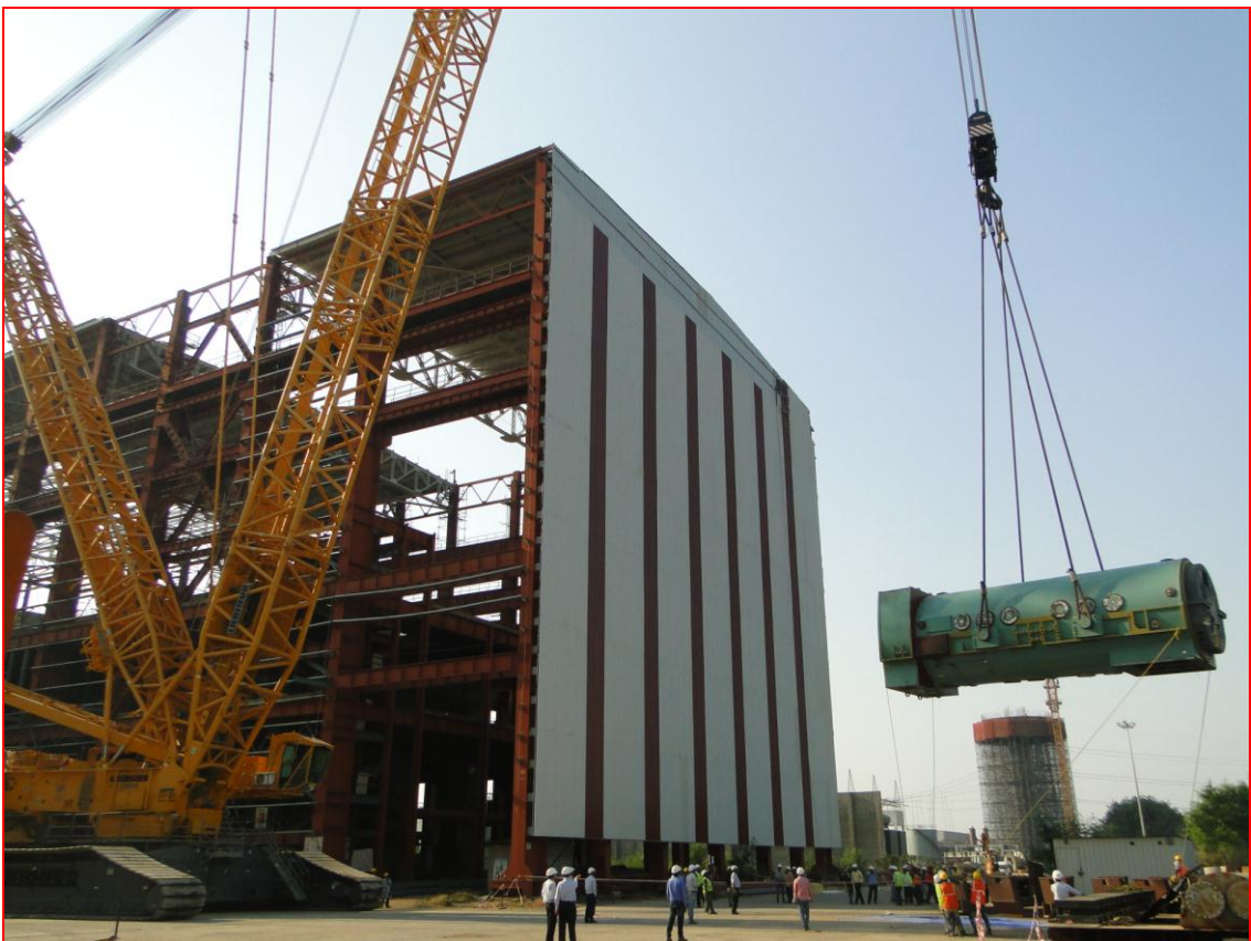
Generator Stator Erection in TB-4
