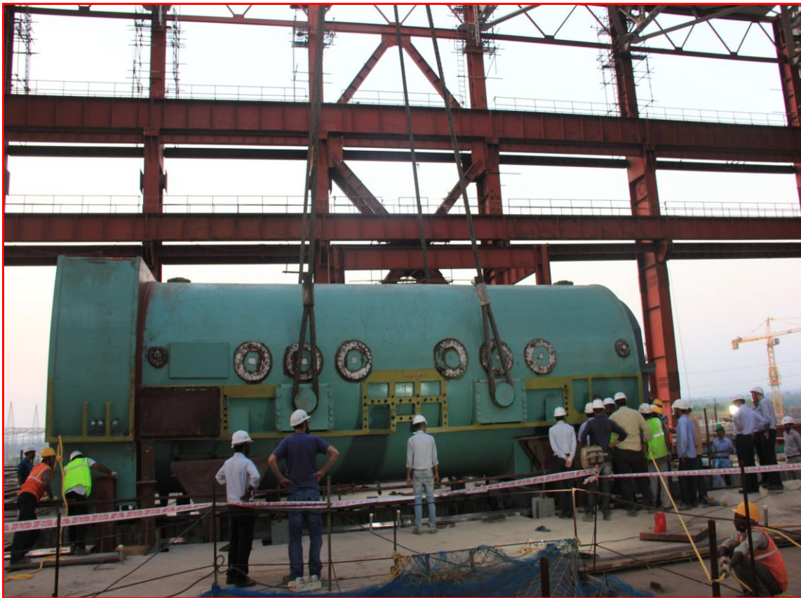
Generator Stator Placement in TG#4 deck at EL 118 M
