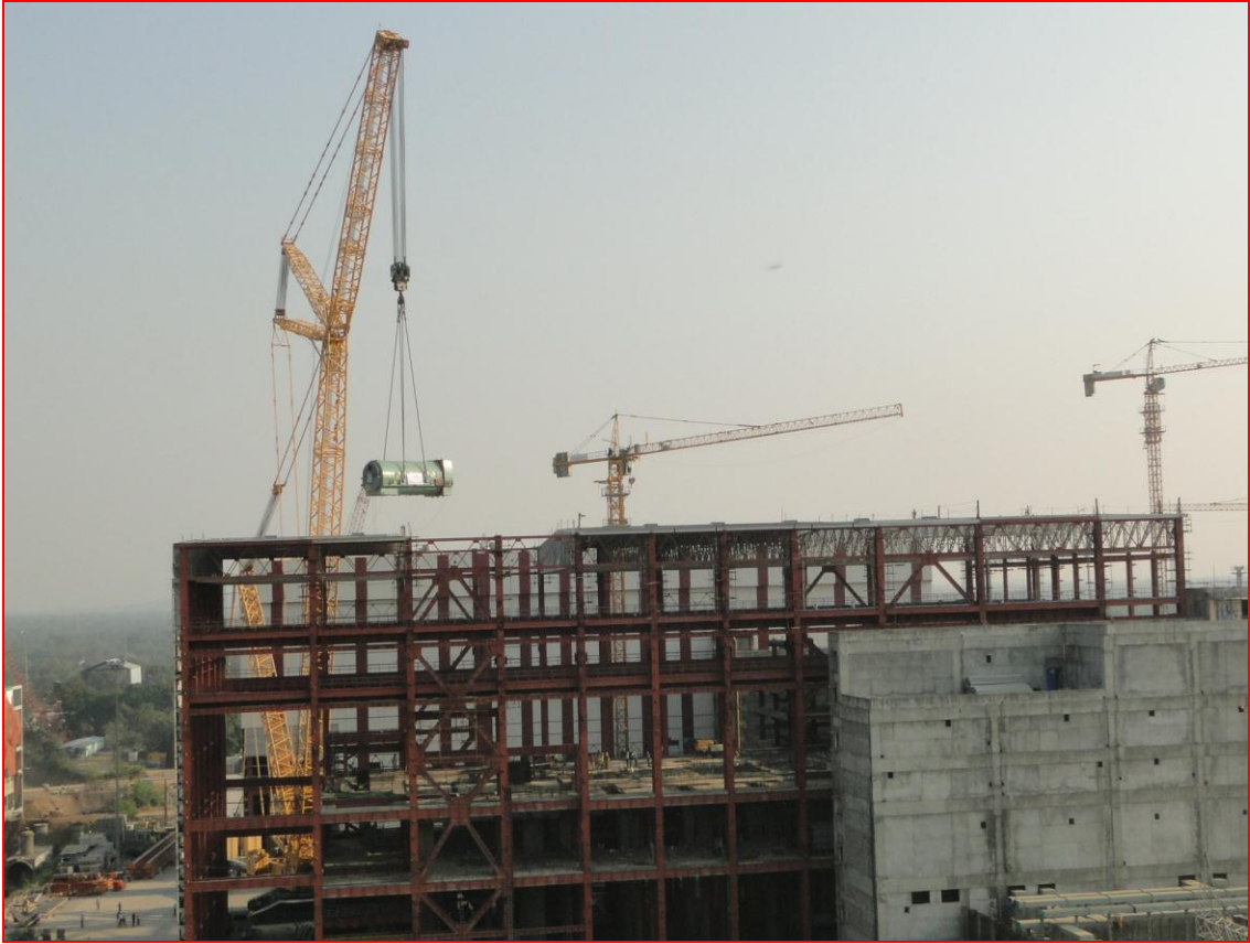
Generator Stator Erection in TB-4
