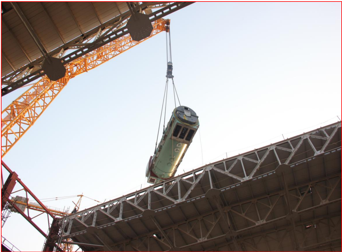
Generator Stator Erection in TB-4
