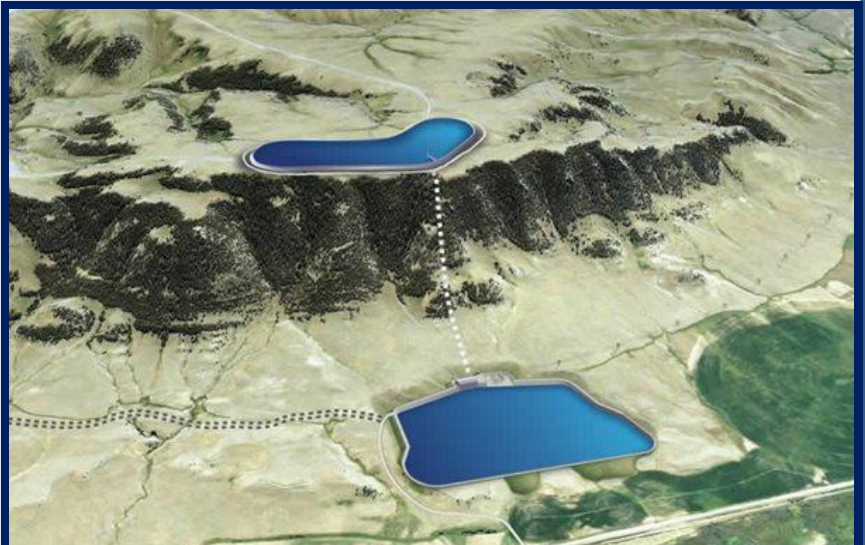
This schematic of the Gordon Butte project is typical of off-river pumped storage (Gordon Butte)
