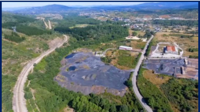
Inside Alpiq's Navaleo pumped storage project in Spain Source: www.waterpowermagazine.com
